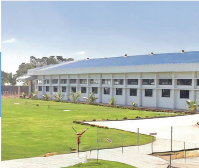
Manufacturing Plant at Nashik, Maharashtra
